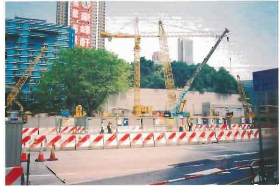
2. PROPOSED MIDDLE ROAD CHILDREN'S PLAYGROUND (LR4) - UNDER CONSTRUCTION
